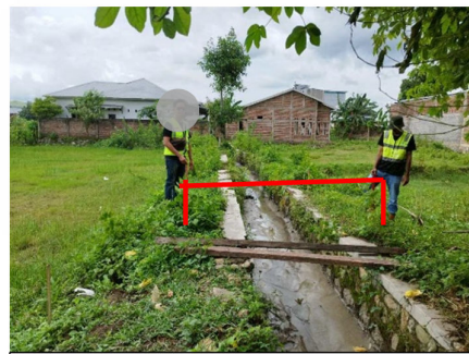
Drainase Primer Rite-Matakando-Santi Lebar eksisting 1,70 m
